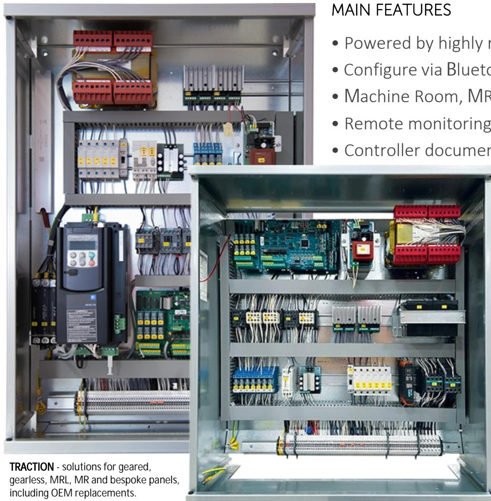
**TRACTION** - solutions for geared, gearless, MRL, MR and bespoke panels, including OEM replacements.
